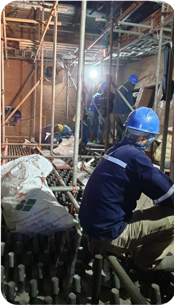
OUTAGE 2019 CLEANING AND INSTALL SCAFFOLDING IN FURNACE
